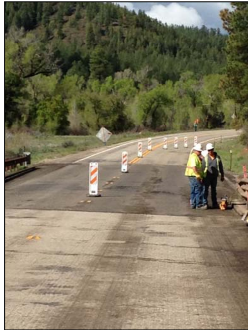
Sawcutting asphalt curb
