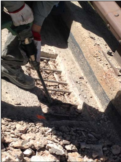
Class II Bridge Deck Repair
