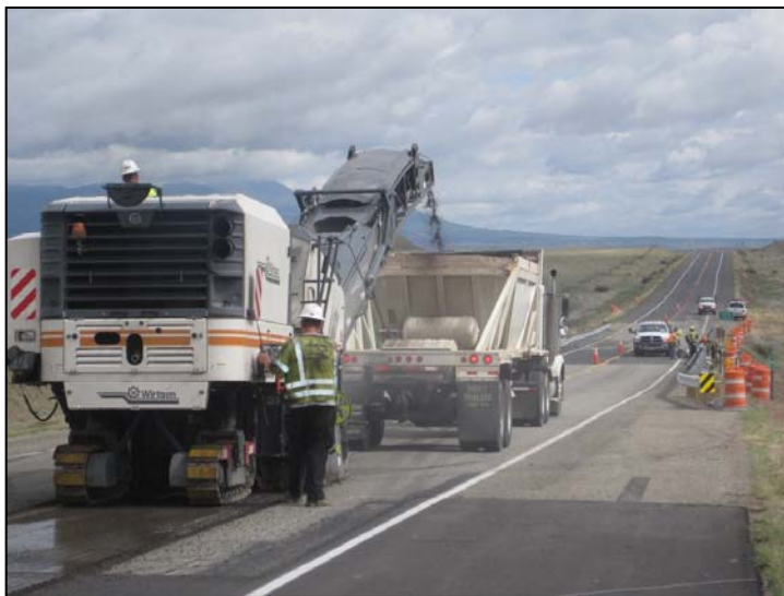
Milling northbound lane at Indian Creek
